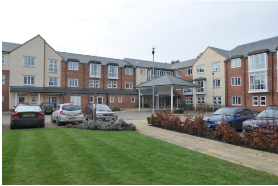
Sunnyfield Lodge Extra Care Housing Scheme, Ripon
